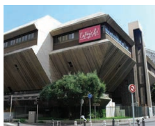
Centre Bourse, Marseille
